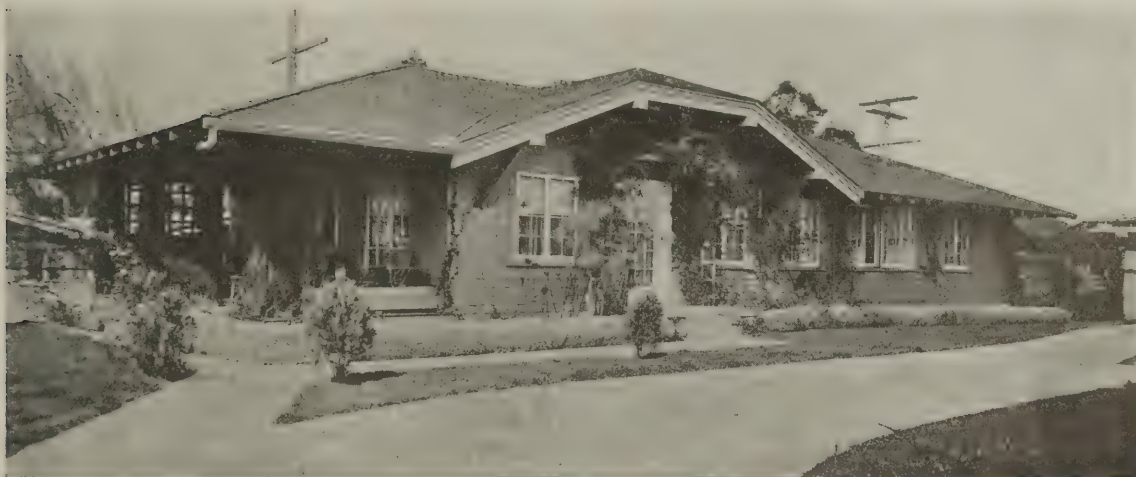
Bungalow at Los Angeles, Cal., designed and built by The Briggs Company
